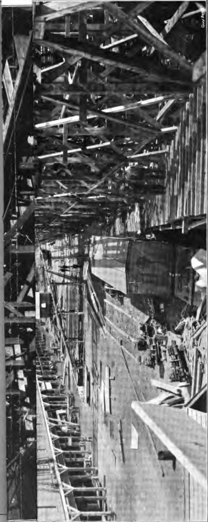
Fig. 4. BROWN GANTRY STEAM CRANE. (AMERICAN S.B. CO., WEST BAY CITY, MICH.)
